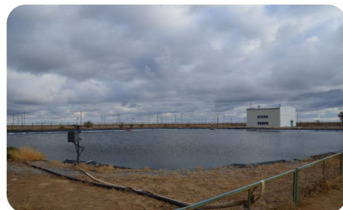
Orталык's wastewater treatment plant
